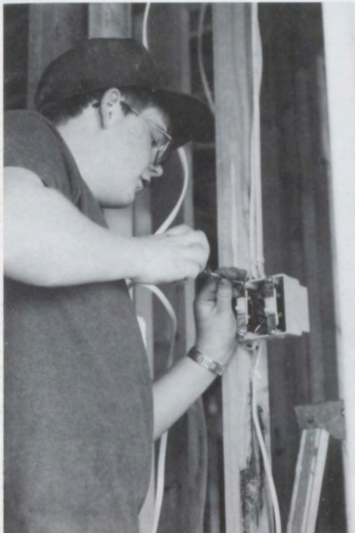
Jason Linne is wiring switches into the house.
