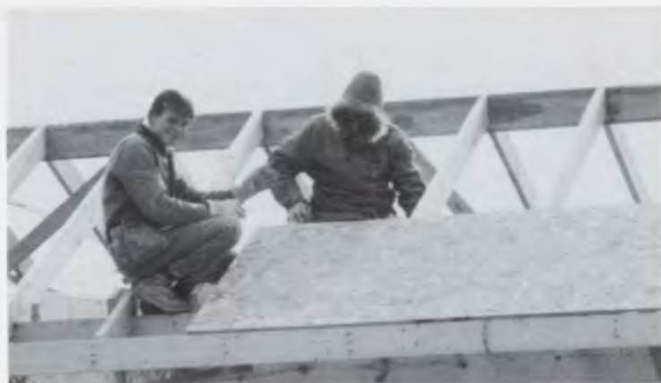
Mike Evrard and Jason Linne are decking the roof on a cold day.
